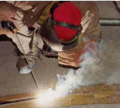
Manual Metal Arc (MMA): High Ni content electrode can be used
